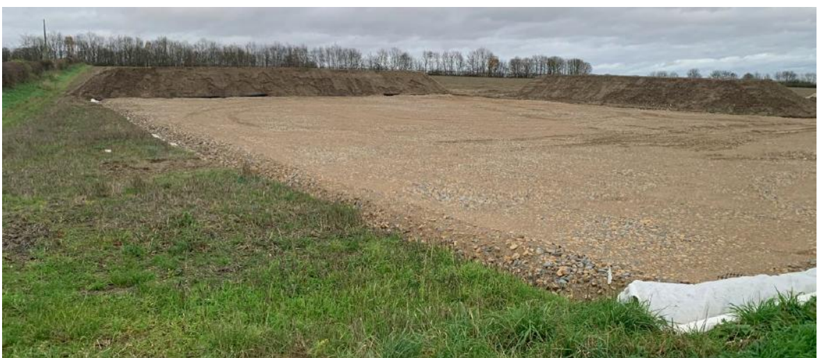
Plate 11-25 Example Construction Compound (being built)
