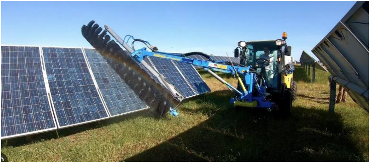
Plate 11-40 Cleaning of Solar Modules
