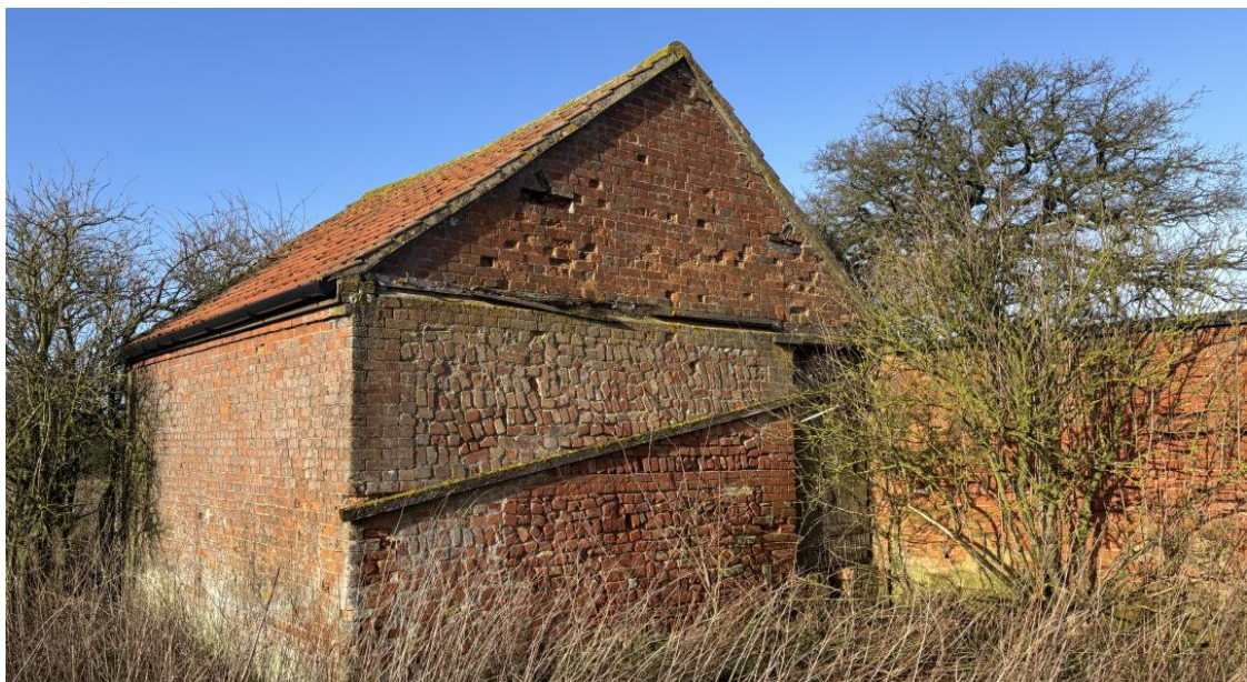
Plate 11-22 Brick Building Within the Site (Field 3)
