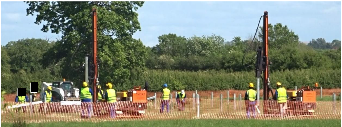
Plate 11-27 Mounting Structure Piles being Installed
