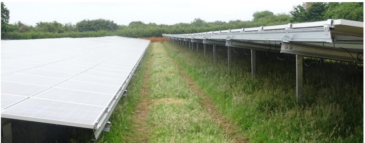
Plate 11-29 Part Installed Panels (Bentham Farm, Purton)
